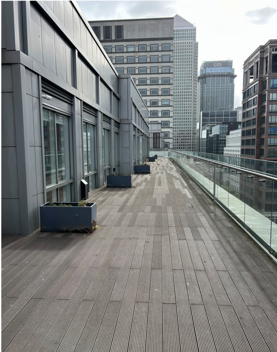
9 th Floor Terrace
