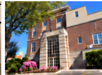
SIDE OF BUILDING
