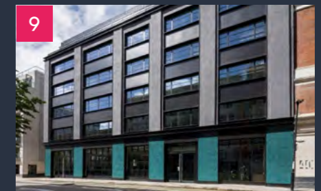
9 SCRIPT, 44 FEATHERSTONE STREET, EC1 Developer LBS Properties Size 44,000 sq ft Use Office Status Completed 2021 - 100% let
