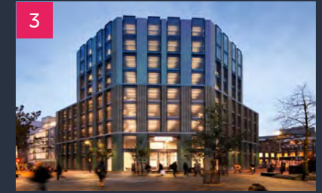
3 DEVELOPMENT HOUSE, 55-64 LEONARD STREET, EC2 Developer CDL Limited Singapore Size 100,000 sq ft Use Office Status Planning granted
