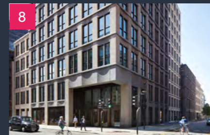
8 THE FEATHERSTONE, 50 FEATHERSTONE STREET, EC1 Developer Derwent London Size 125,000 sq ft Use Office Status Completed 2022 - 92% let
