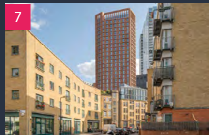
7 39-47 EAST ROAD, N1 Developer Aviva / Summix ERL Size 23 storey Use Hotel & 60,000 sq ft of office Status Target completion Q4 2024
