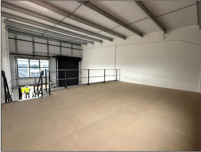
First Floor of a half Mezzanine Floor Unit
