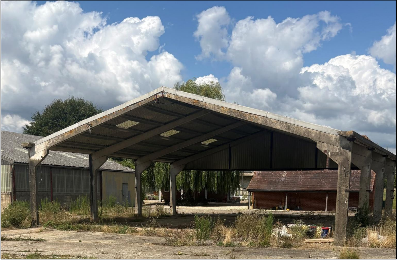
Adjacent open sided Atcost barn
