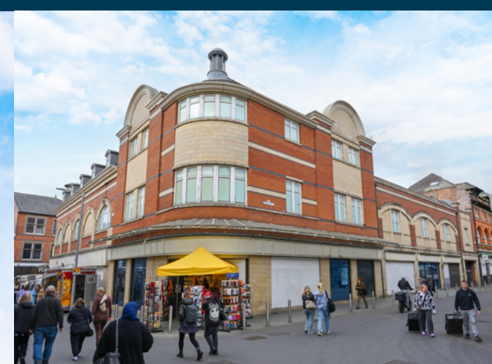
Above: Lincoln St and Clinton St West frontage
