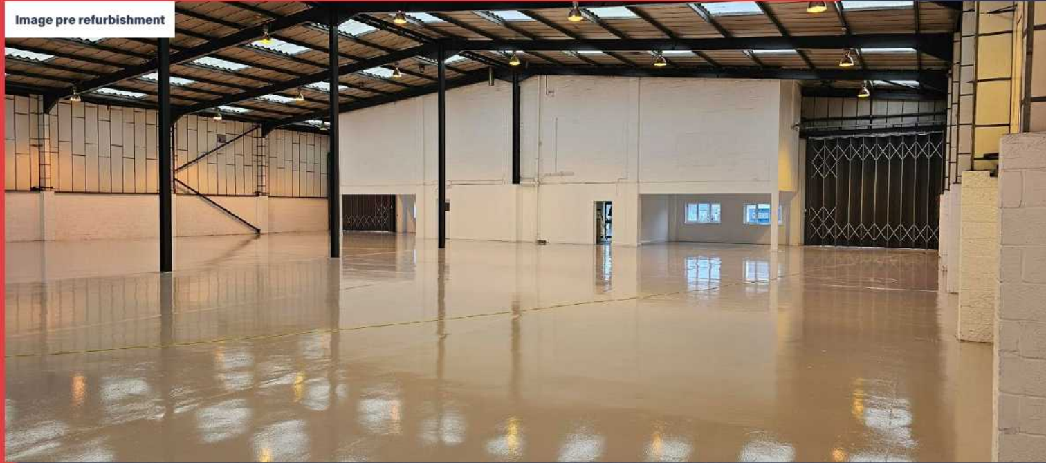
Image pre refurbishment
