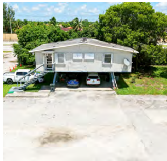
1,500 SF ELEVATED OFFICE
