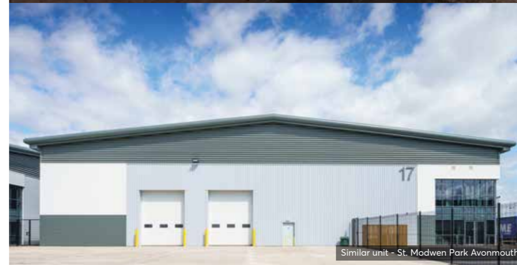
Similar unit - St. Modwen Park Gloucester
