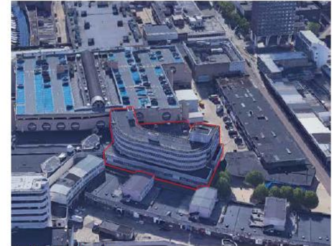
Aerial view looking West
