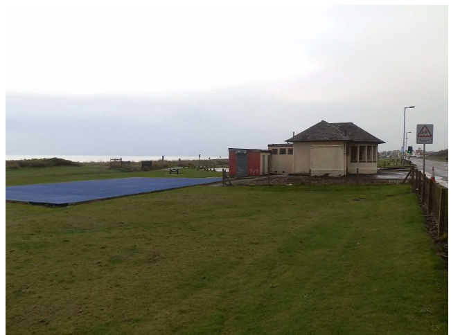
3. VIEW FROM SOUTH SIDE
