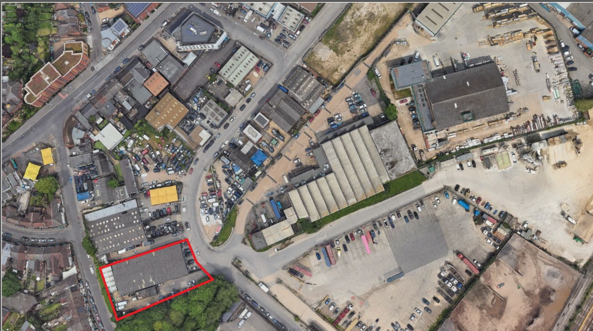
Aerial Imagery – Site Extent (rear small unit will be removed)
