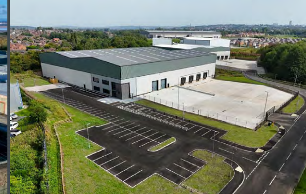
Cobalt Park Oldham Broadway Business Park Chadderton
