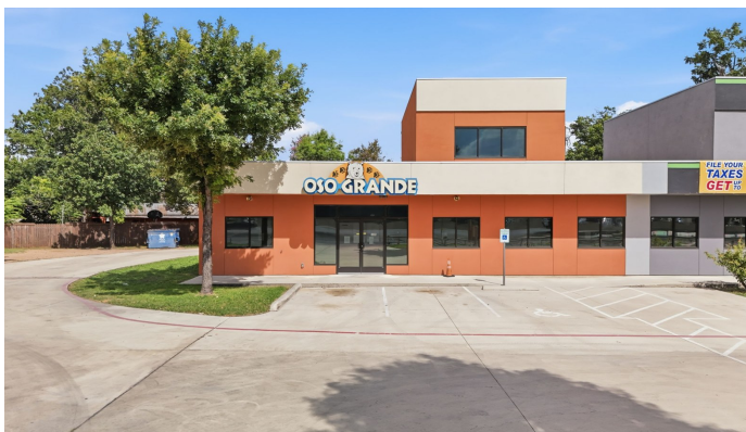
Building frontage and customer parking
