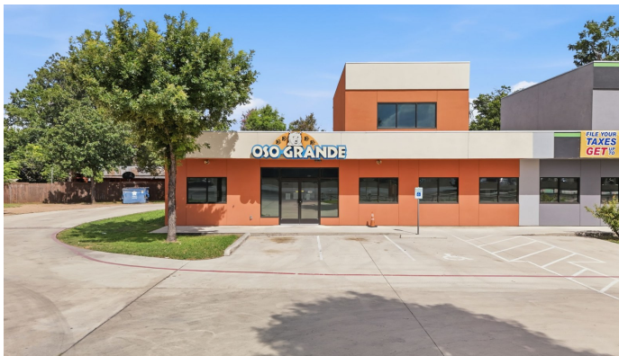
Building and gated approach
