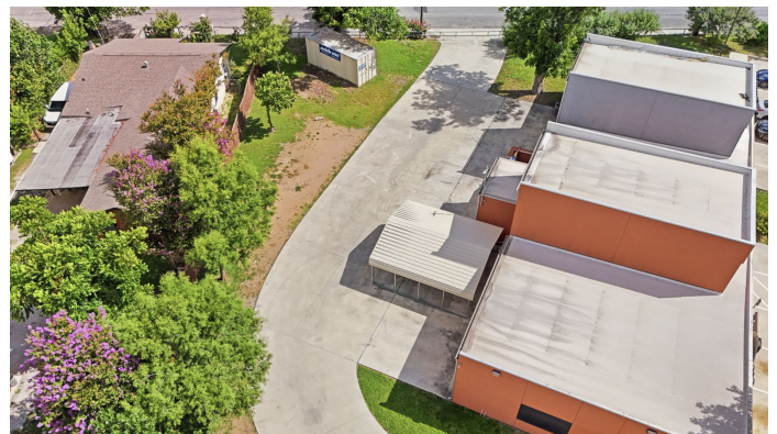
Overhead view of building, canopy and paved yard
