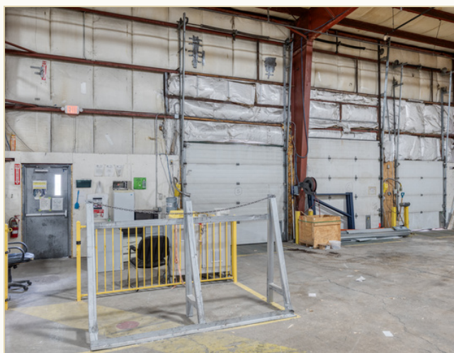
UTILITY / DOCK SUPPORT AREA
