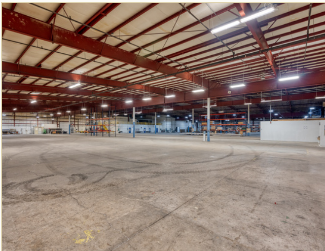
OPEN WAREHOUSE FLOOR
