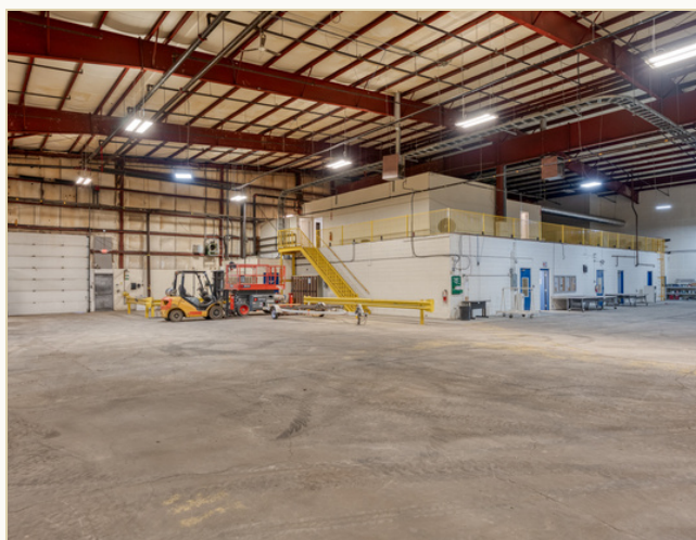
WAREHOUSE FROM MEZZANINE
