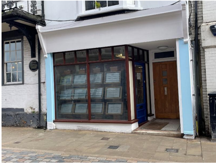
Front entrance to shop and flat 49c
