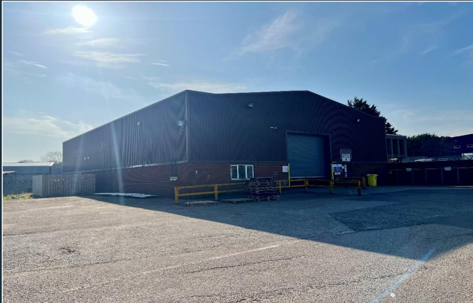
External of Building 1
