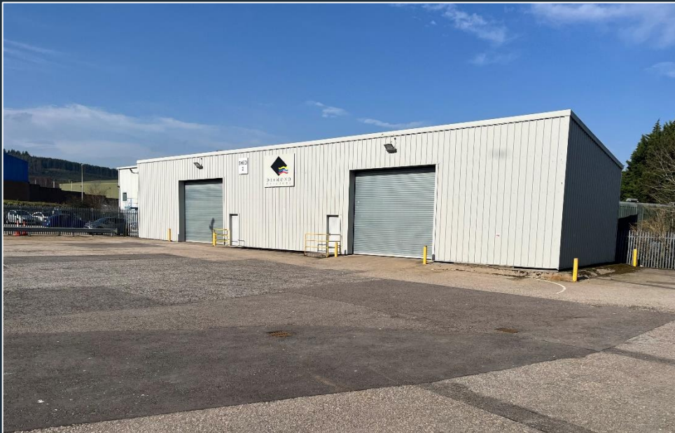
External of Building 2
