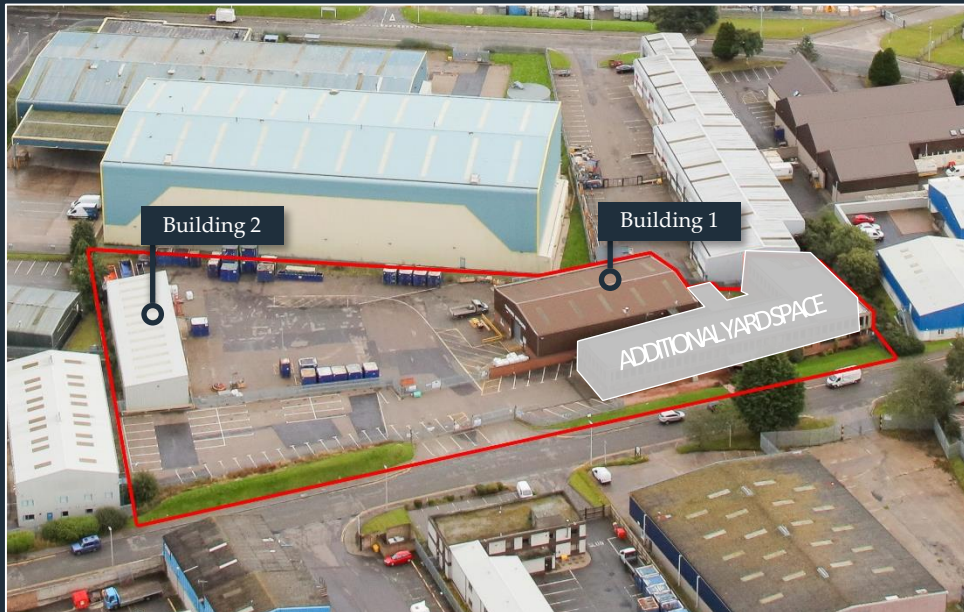
Building 1 and 2 are available in whole. The existing office accommodation is to be demolished.
