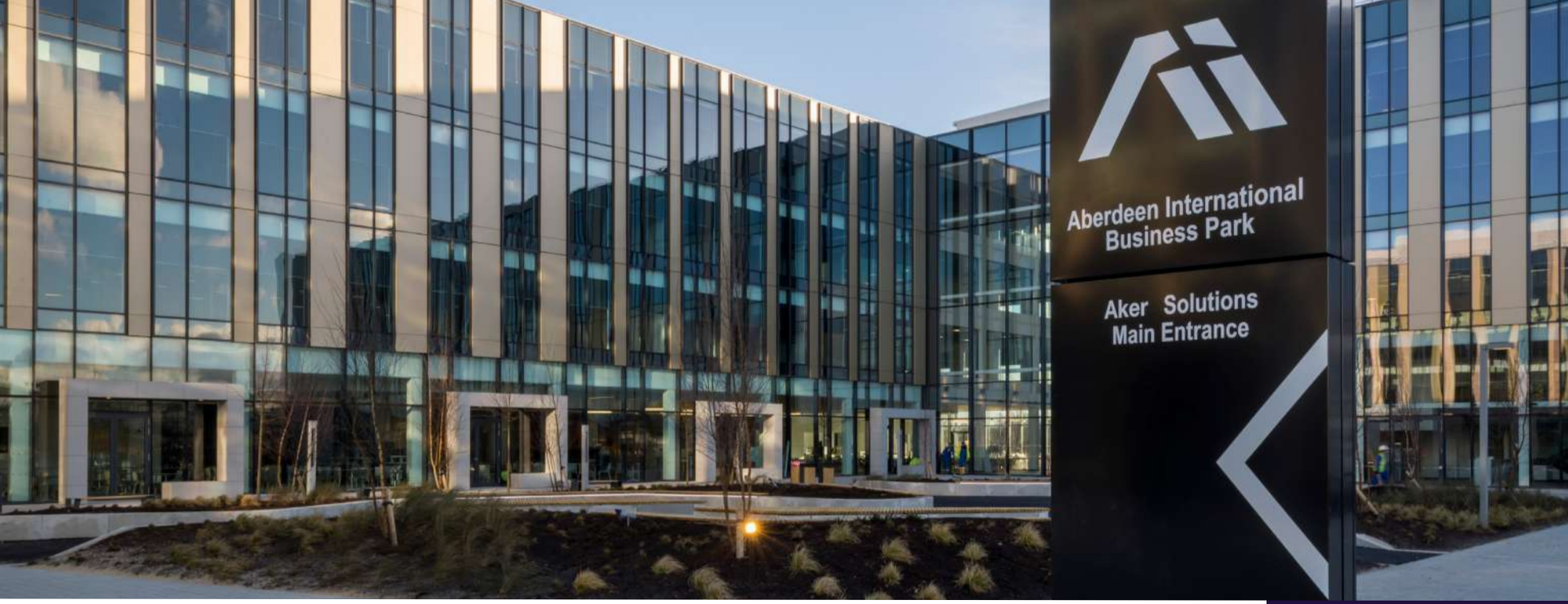
Aberdeen International Business Park (AIBP)
