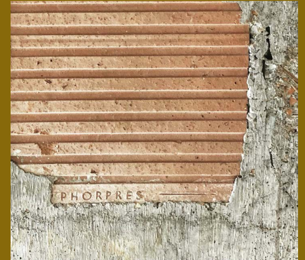
EXPOSED HOLLOW POT SOFFIT
