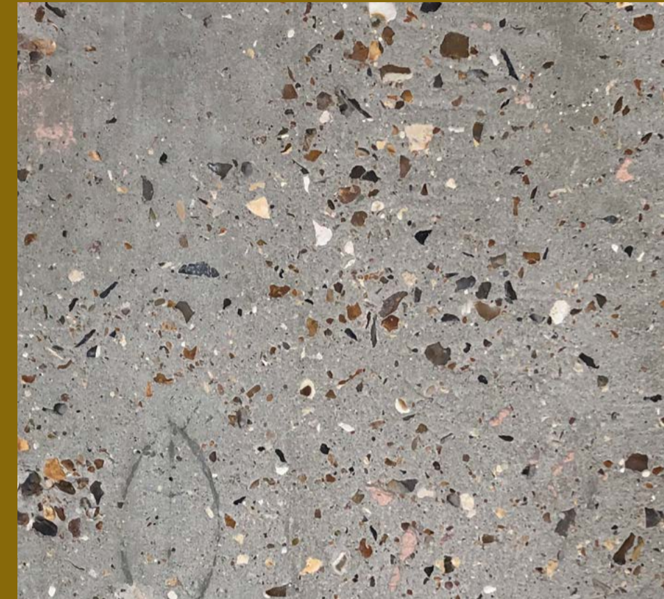
EXPOSED CONCRETE STRUCTURE
