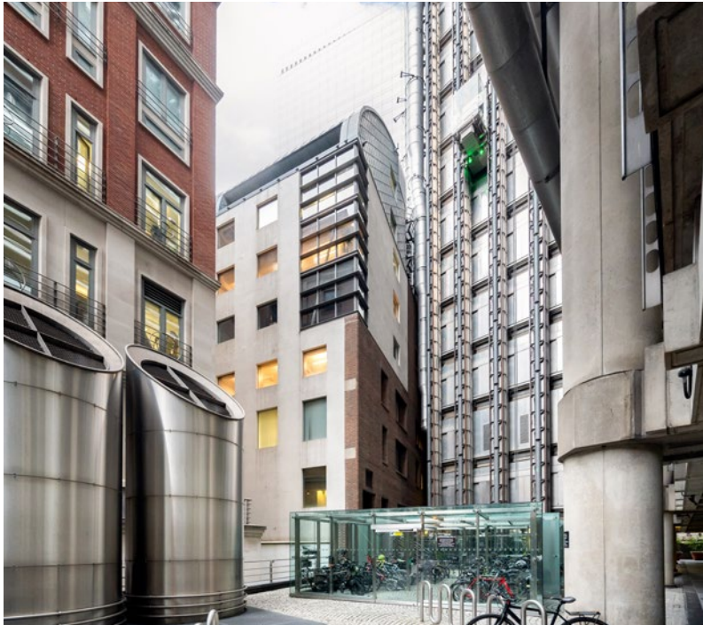
South and east elevations of 11 Leadenhall Street
