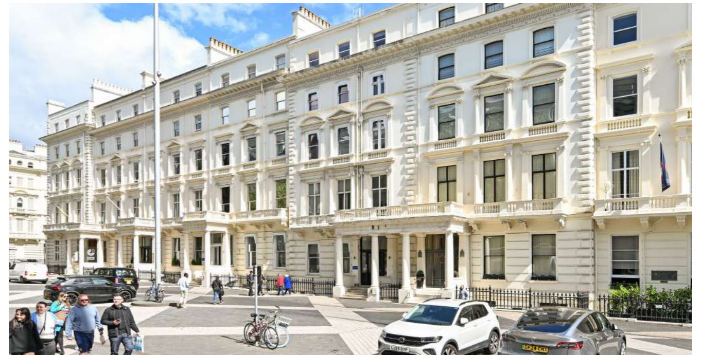
View over Prince's Gardens from the private rear terrace
