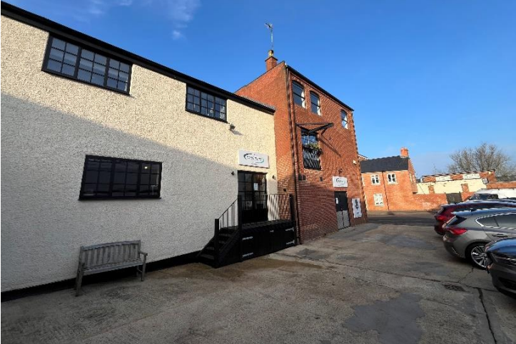
Rear Office and Parking
