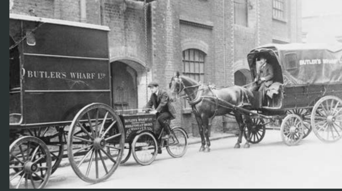
Carriages from Butlers Wharf Ltd
