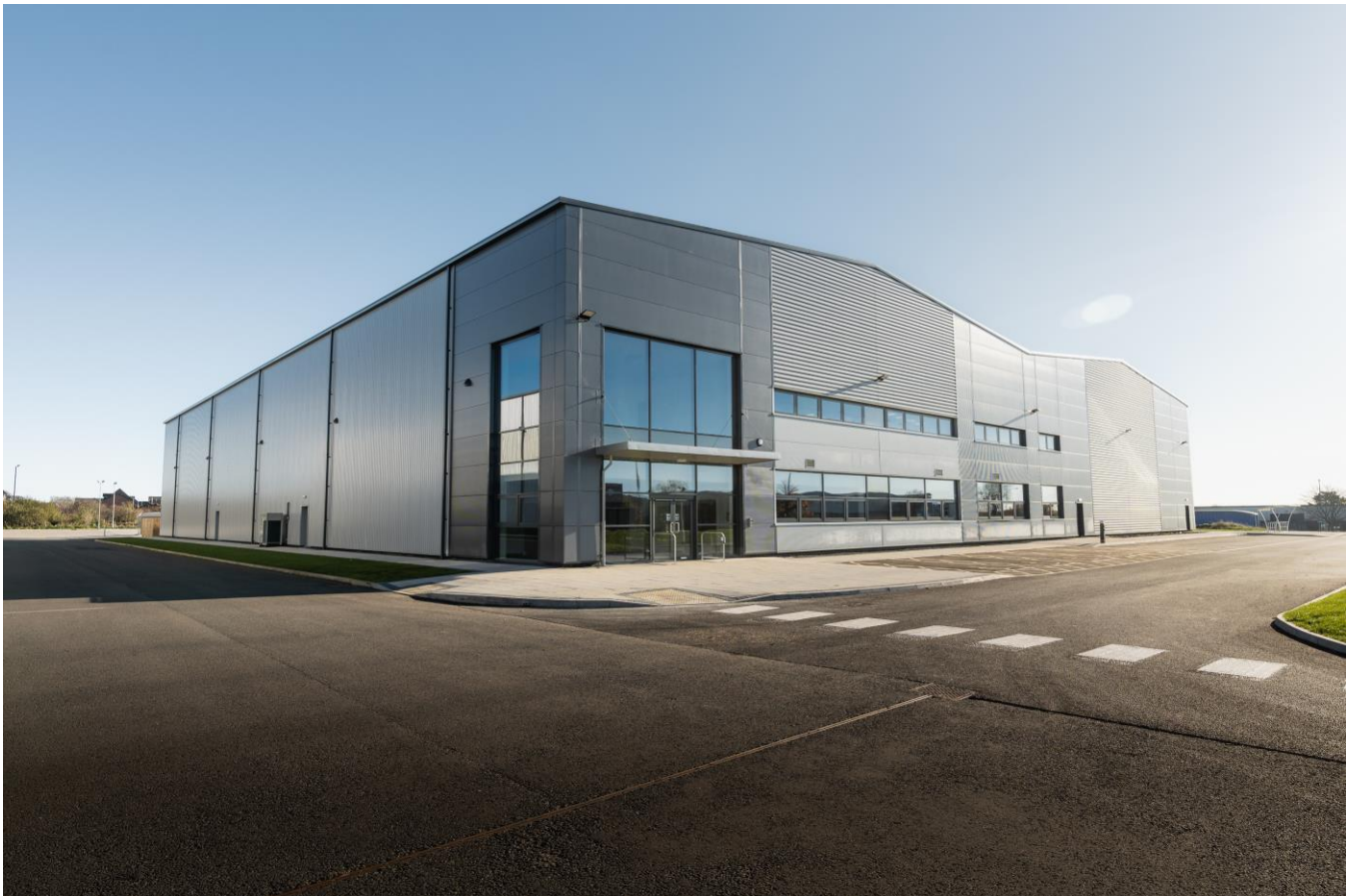
Image of completed Unit L6 (June 2023)
