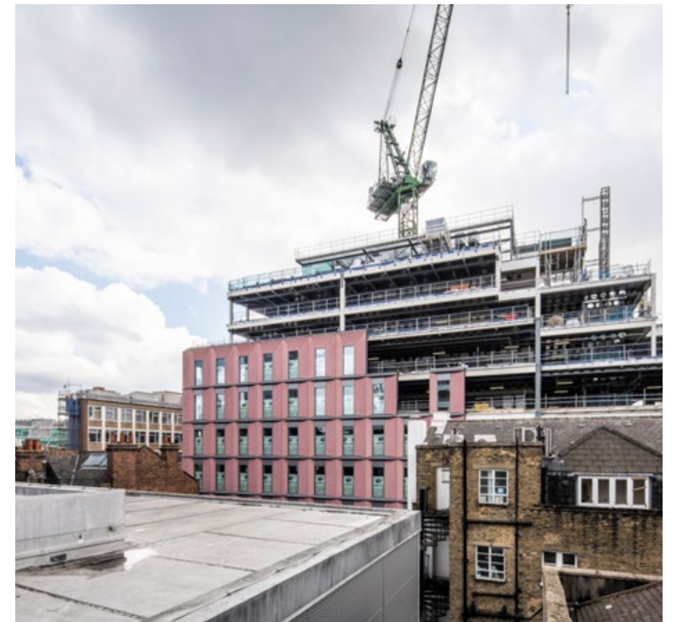
Significantly under-developed site in context of surrounding schemes
