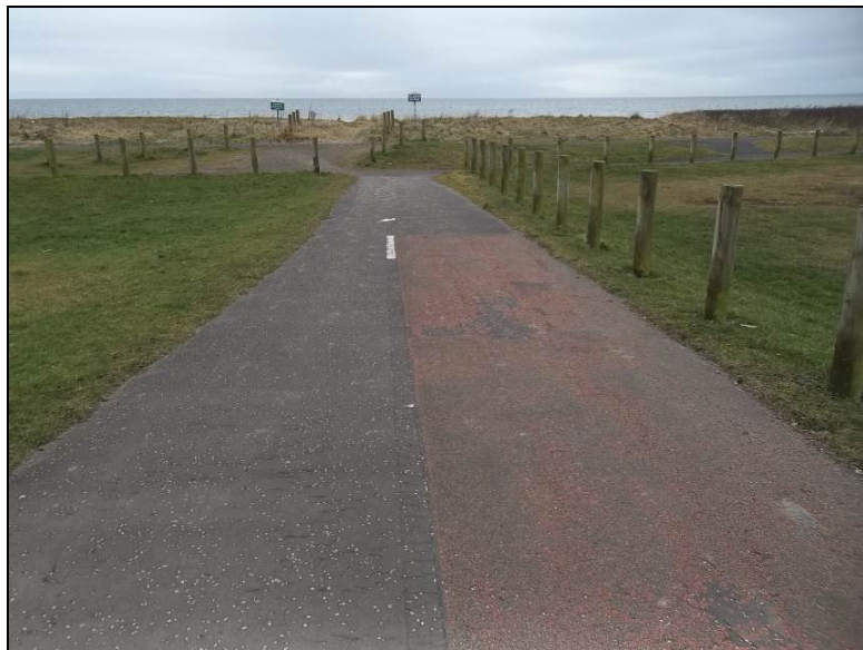
Shared Footpath/ cyclepath link from signalised pedestrian crossing of Beach Road
