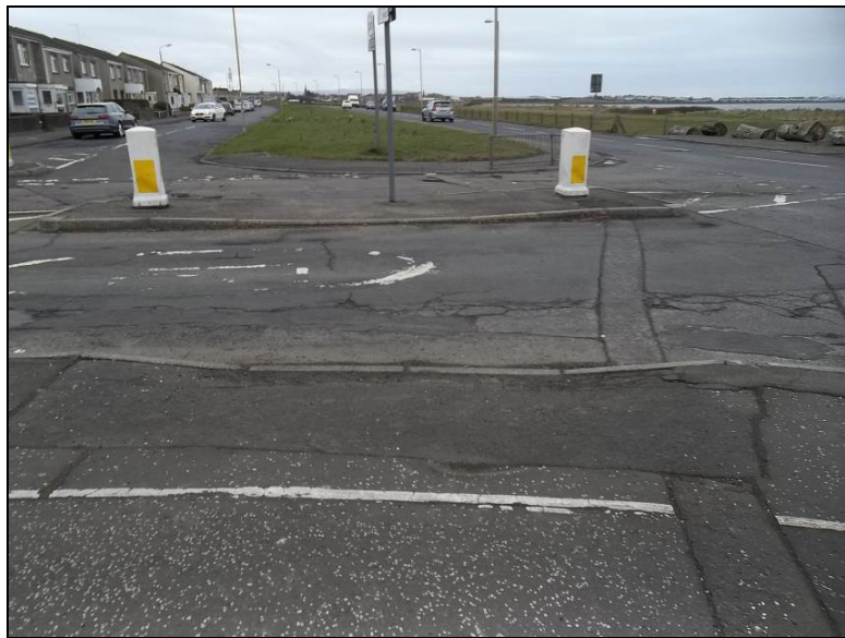
Uncontrolled pedestrian crossing of Burnfoot Avenue at Beach Road, with dropped kerbs, looking south
