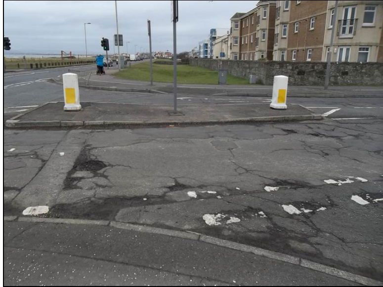
Uncontrolled pedestrian crossing of Burnfoot Avenue at Beach Road, with dropped kerbs, looking north
