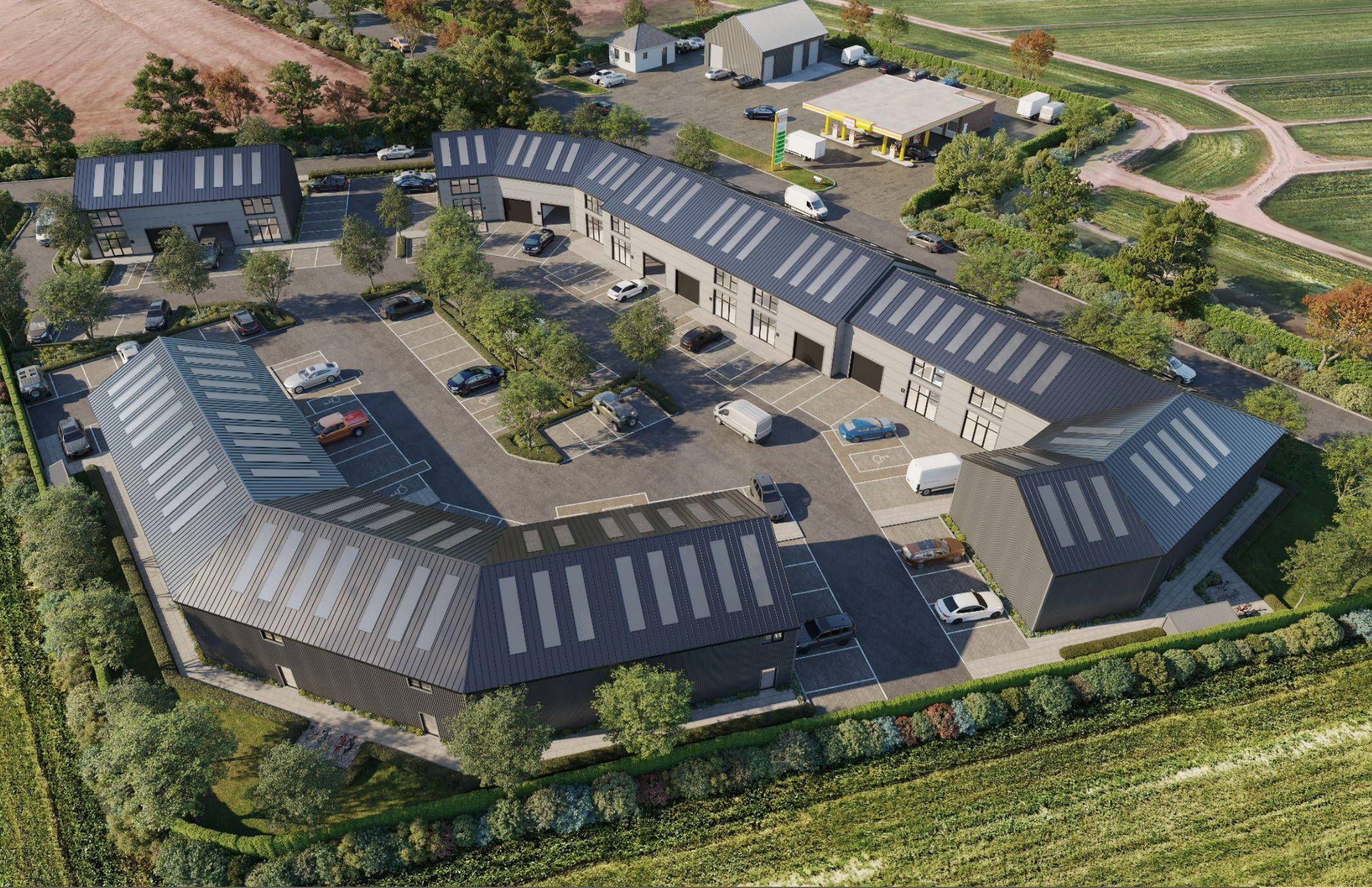
Aerial CGI of Apollo Business Parks at Souldrop | 14 NEW BUILD FREEHOLD COMMERCIAL UNITS
