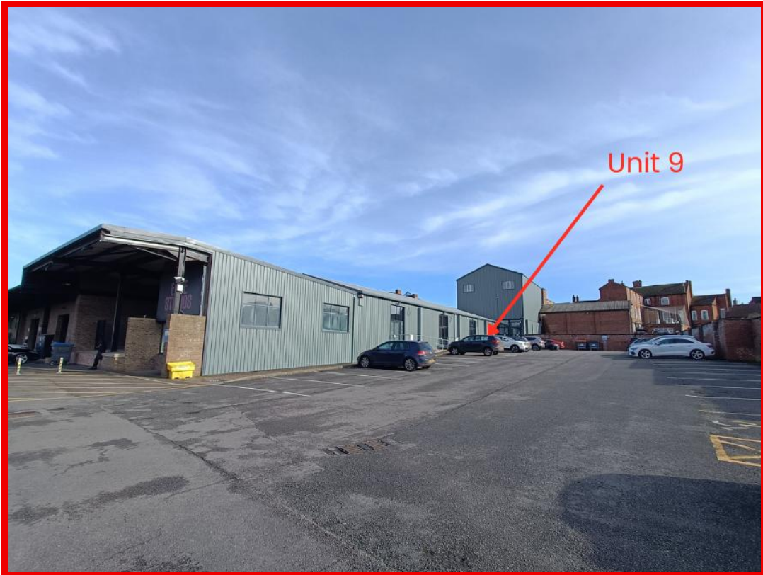
Chandlers Yard Business Park car park
