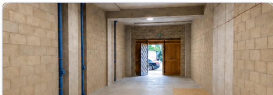
Ground floor - view towards street
