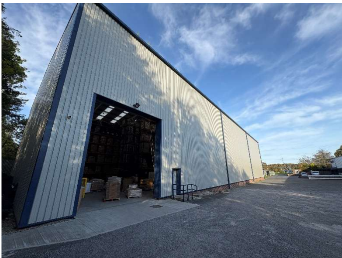
Unit 2 High Bay Warehouse
