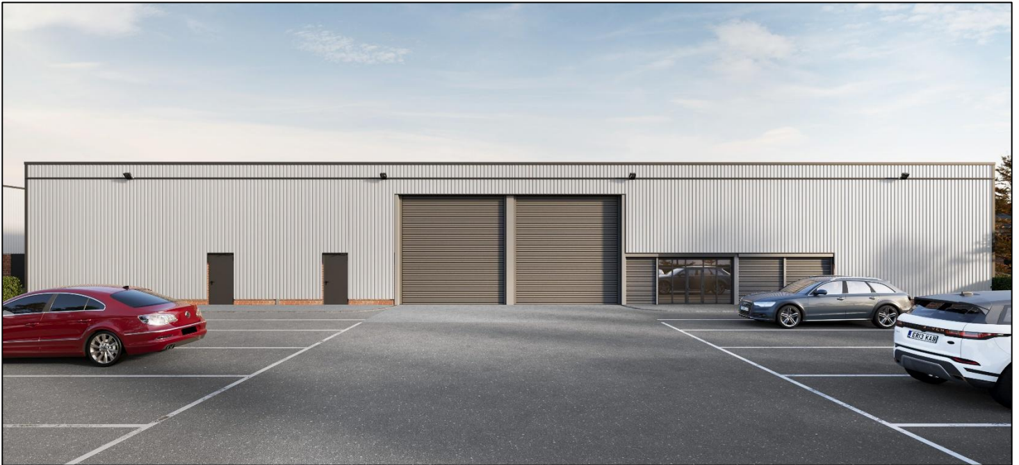
CGI showing unit post refurbishment
