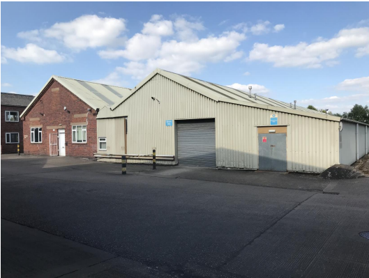
Unit F and Western Entrance of Main Unit
