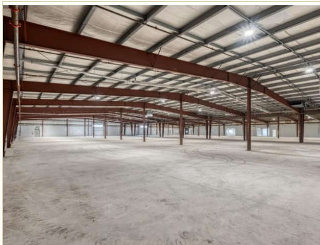
OPEN WAREHOUSE FLOOR
