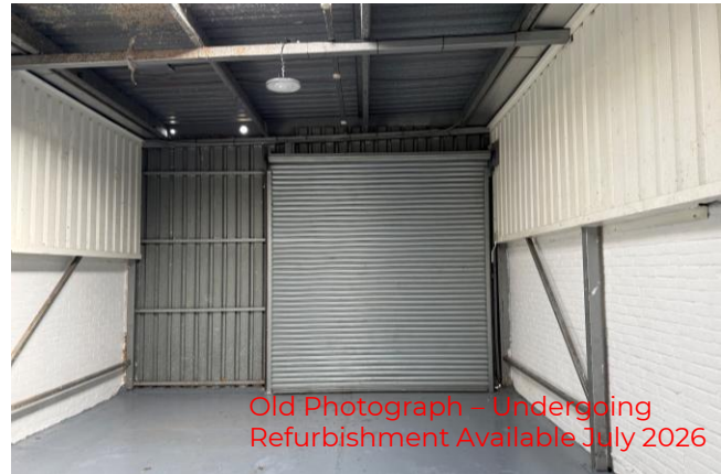
Old Photograph – Undergoing Refurbishment Available July 2026
