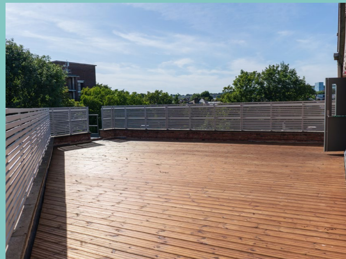
WAREHOUSE - 2ND FLOOR TERRACE
