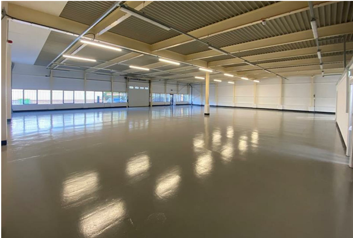
Pictures from initial refurbishment
