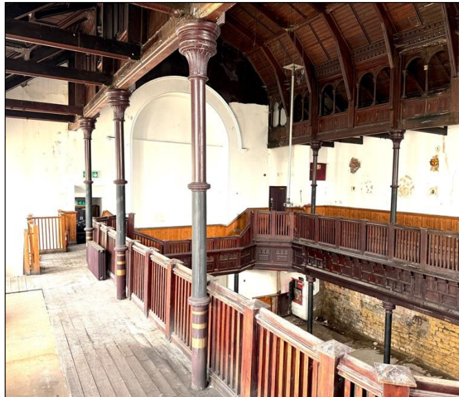
Internal – First Floor
