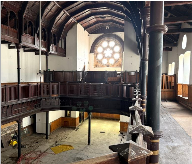
Internal – First Floor
