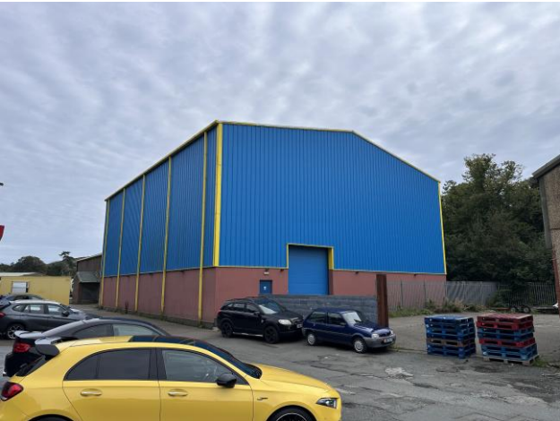
Extension warehouse – large eaves height
