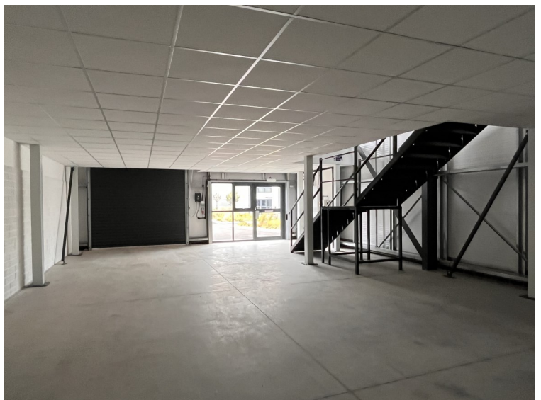
Ground floor prior to fit-out
