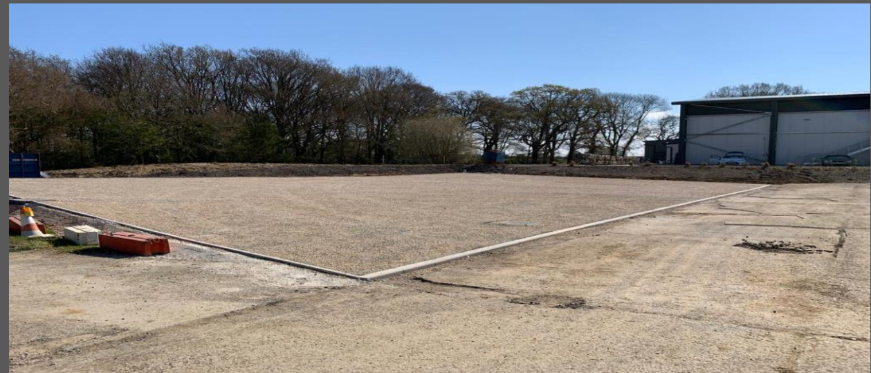
Example of Parking Surface
