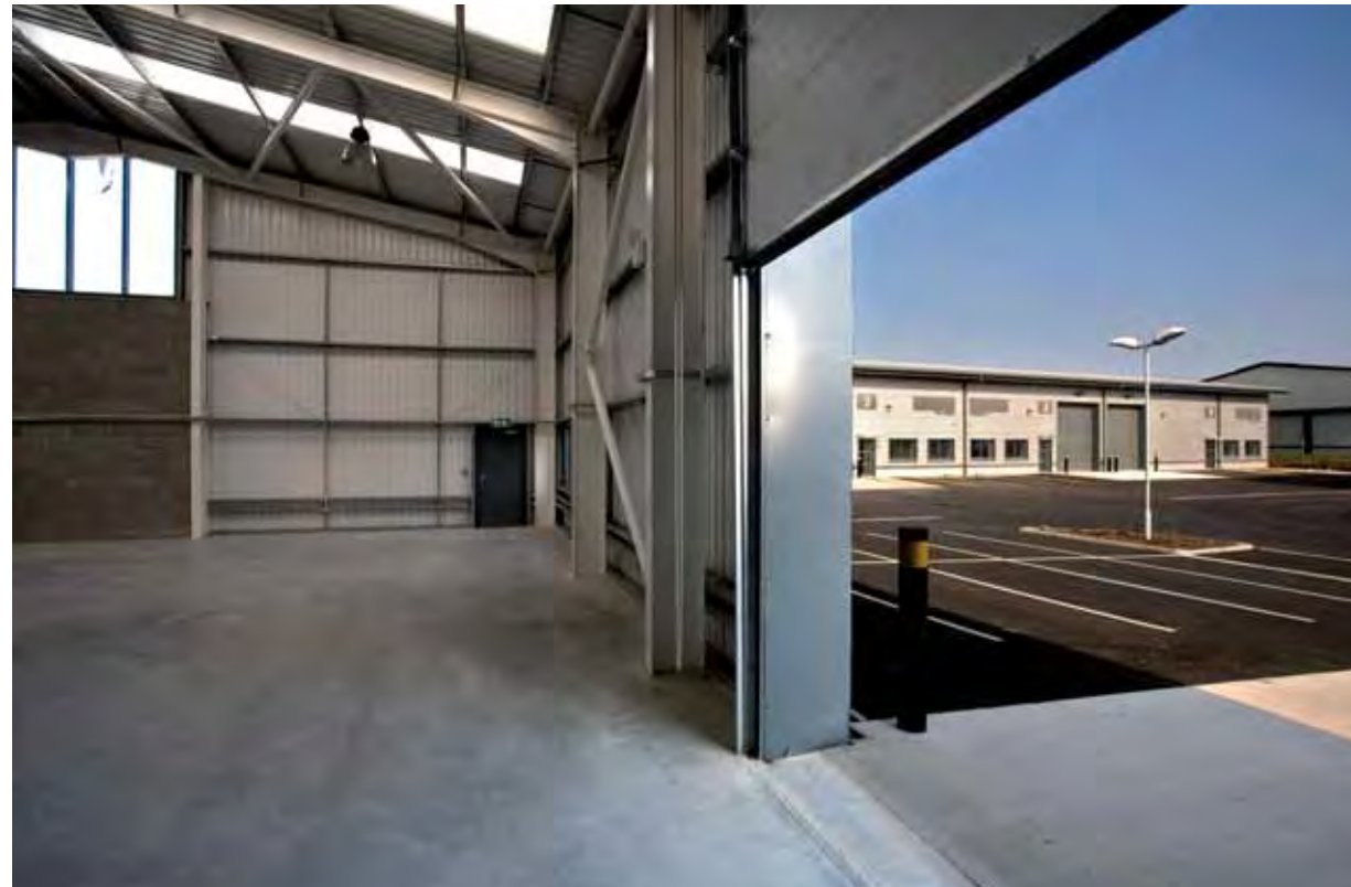
■ Warehouse Access - Unit 14
