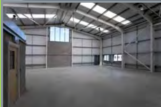
■ Typical Unit Interiors
