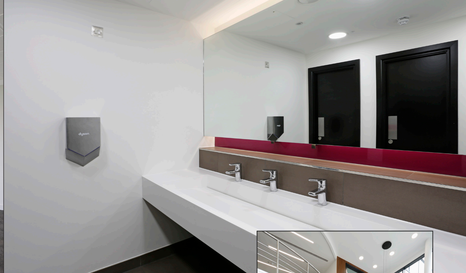
Showing finishes post refurbishment
