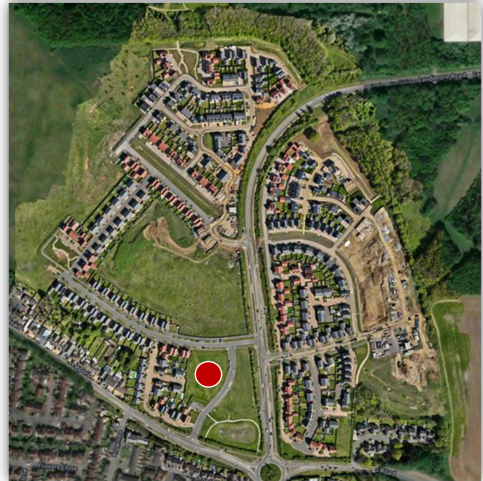
The above is an aerial image of Phase 1 (April 2026), illustrating construction progress, with the local centre parcel now largely surrounded by occupied dwellings
